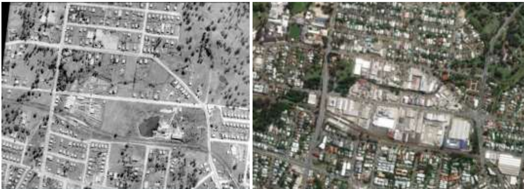
Figure 1 Channelisation and floodplain encroachment by commercial development near Grinstead Park. Historically meandering channel within a broad floodplain in 1936 (left image). Straight concrete channel with a constrained floodplain in 2023 (right image).
