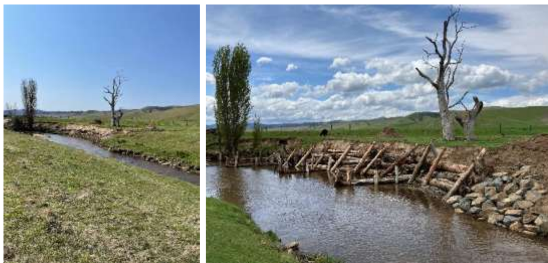
Figure 5 Pre (L) (2023) and post (R) (April 2026) image of Habitat work for Macquarie Perch on Livingstone Creek, Omeo
