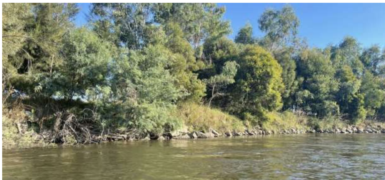
Figure 2 Bank restoration works (rock revetment and riparian revegetation) along the Upper Murray River (T. Wallis, RMCG, 2024)
