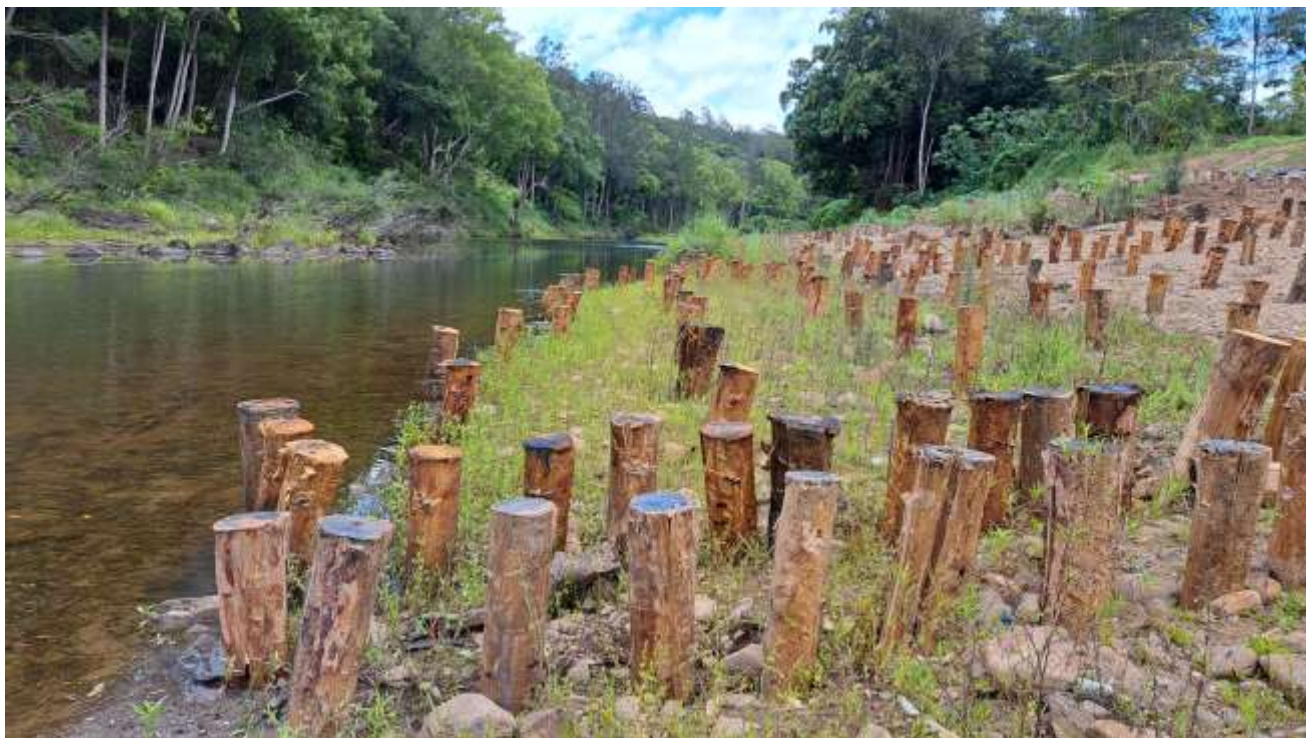
Figure 1 Example of riverbank stabilisation works on the mid-Tweed River (December 2023)
