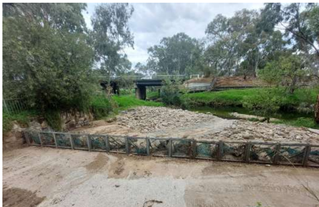
Figure 2 GPT at Third Creek and River Torrens confluence
