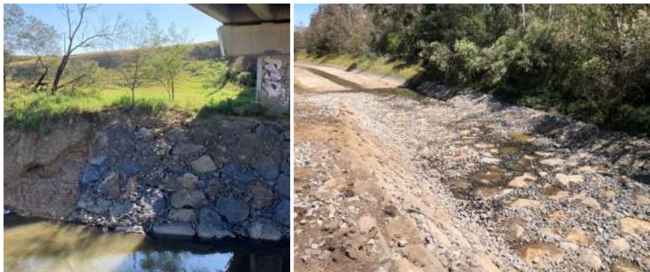
Figure 1 Waterway rock installations showing use of predominately single sized rock, placed to create a smooth surface and infilled with small gravels. LHS image also shows bank slope significantly steeper than 2H:1V
