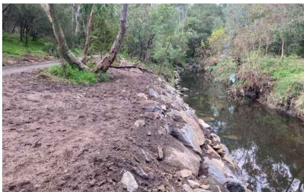
Figure 2 Waterway bank protection rockwork showing use of predominately single sized rock, slope steeper than 2H:1V and building-out into channel
