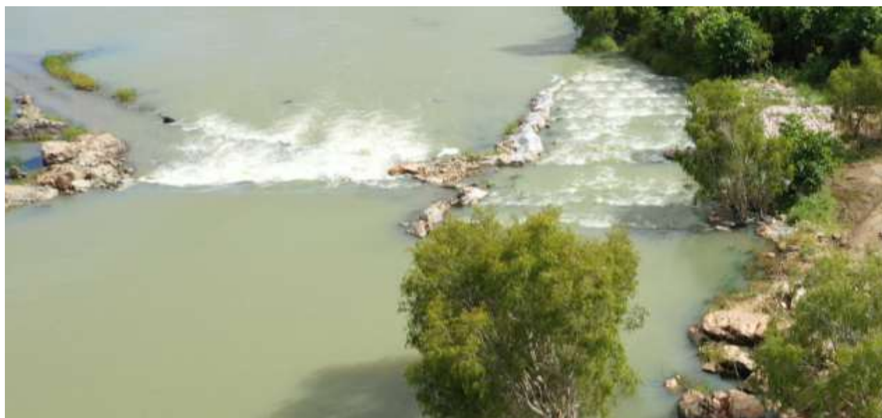
Figure 2 Warrens Gully – rock-ramp fishway
