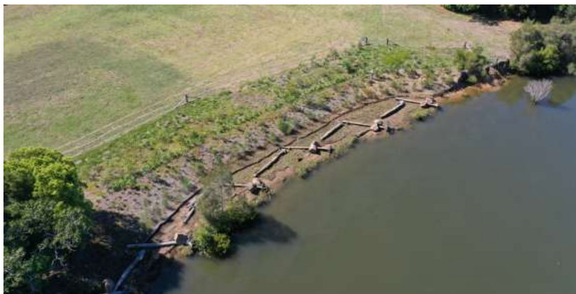
Figure 1 Site B1 showing the intertidal bench with rootball logs and plain logs arranged to break up boat wash and provide a sheltered environment for mangrove establishment. Construction winter 2023. Photo September 2024
