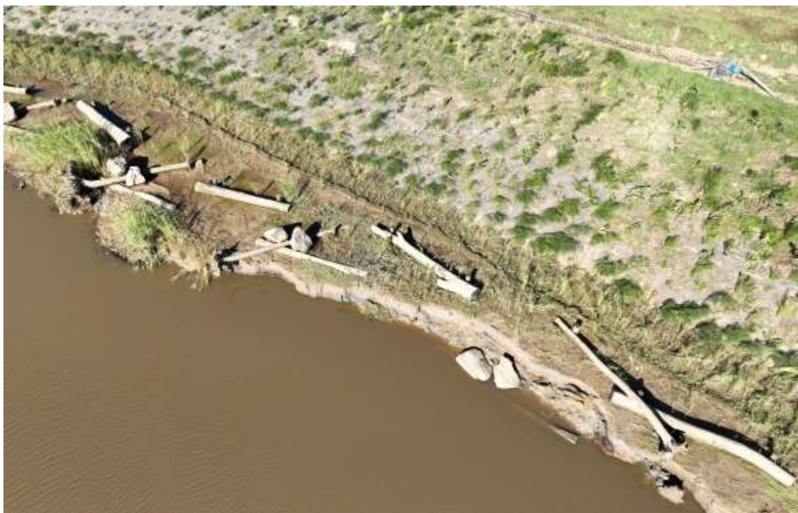
Figure 5 Site 24 showing bench as constructed (left of image) and a section of severe bench erosion and log movement (right of image). In this location, the restoration is considered unsuccessful as there is very limited remaining intertidal zone to support future establishment of a resilient mangrove fringe. Photo March 2025 (post flood), following construction winter 2024
