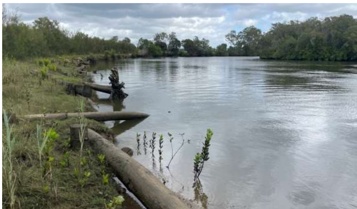
Figure 3 Site 5 showing an area with log rotation, loss of boulders and modest bench erosion. This area is still progressing consistent with the design intent. Construction Spring 2023. Photo May 2026
