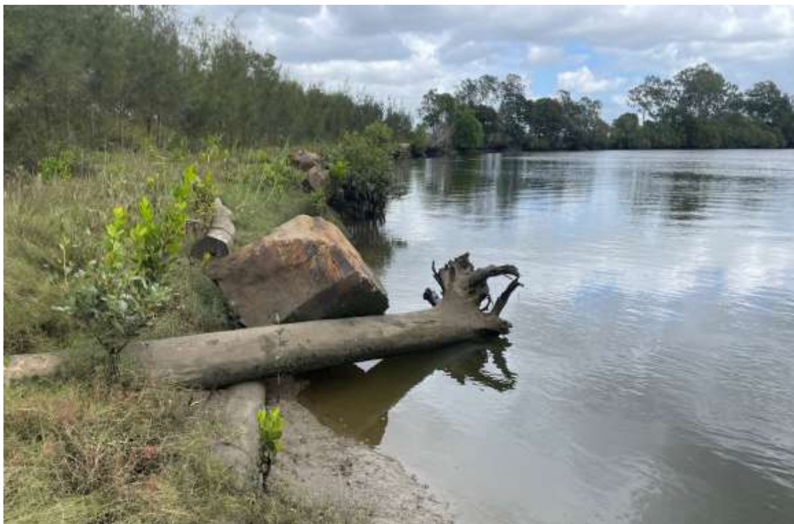
Figure 4 Acceptable bench adjustment. One boulder dislodged, but the rootball remains in contact with flow. Complete groundcover of intertidal vegetation, with mangrove saplings growing slowly. This site is progressing consistent with the design intent. Photo May 2026. Construction Spring 2023
