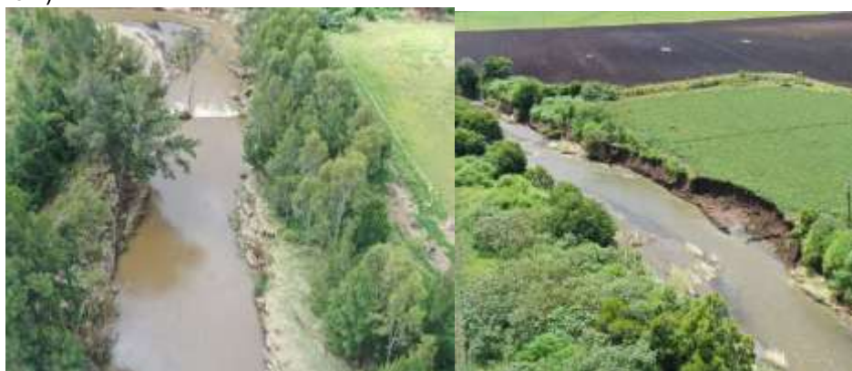
Figure 4 Aerial photos post Cyclone Alfred (March 2025) - Left -2017 stabilised bank, Right - untreated bank
