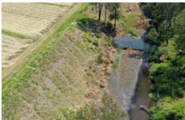
Figure 2 Cross channel structure looking downstream, with sediment deposition upstream and the formation of a bench that is commencing to revegetate (08/10/2024)
