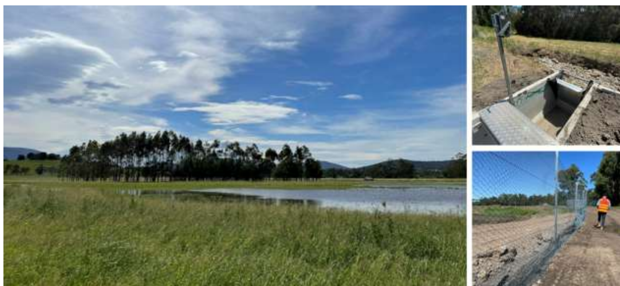
Figure 7 Photograph of constructed seasonal wetland on Birrarung floodplain, creek diversion structure and herbivore exclusion fence. Vegetation planting is planned to be undertaken between August and December 2026
