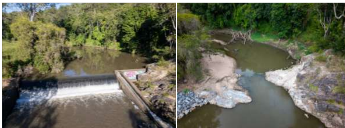
Figure 2 Before and after removal image of Luscombe Weir location, Albert River
