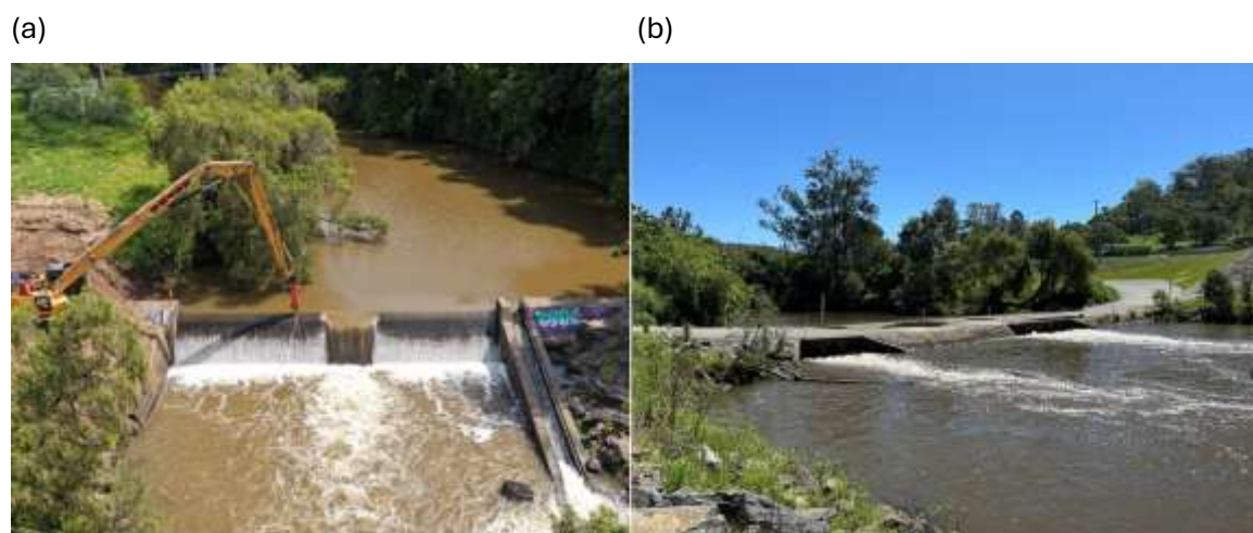
Figure 6 (a) Demolition commencing on Luscombe Weir, November 2025; (b) Stanmore Road Causeway, Yalata. The last remaining waterway barrier on the Albert River, Qld. It is scheduled for removal in 2026
