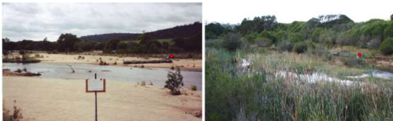
Figure 3 Site of large wood installation in the Genoa River floodplain reach in 2002 (left) and 2009 (right). Note the establishment of in-stream vegetation and development of a narrow low flow channel
