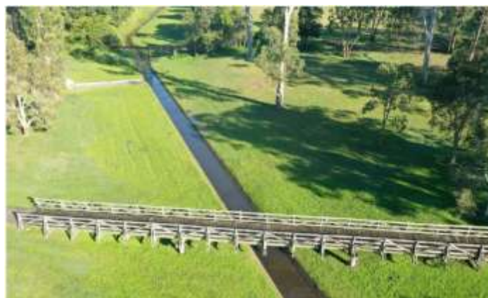
Figure 6 Concrete channel that will be naturalised as part of the co-funded project in Slacks Creek
