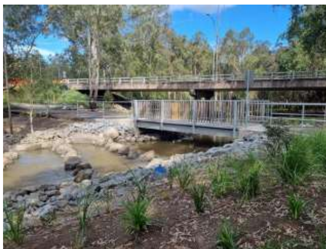
Figure 5 Queens Road fishway and pedestrian bridge to replace aging and inappropriately sized culverts for the previous pedestrian bridge. Delivery of this infrastructure included a rock fish ramp so support fish passage
