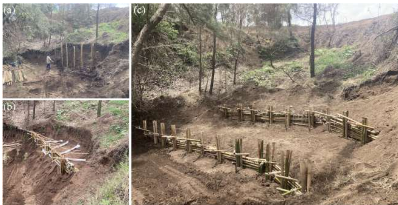
Figure 4 Bamboo retaining wall. Construction stages showing (a) the vertical bundles placed into the pre-drilled holes just before being driven one meter deeper – stack of bundles are visible on the ground. (b) Completed top retaining wall including piles, sleepers, tiebacks and drains all made of bamboo, before backfilling. (c) Completed wall
