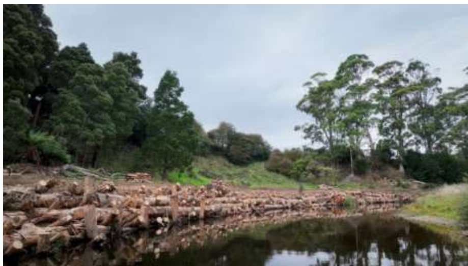
Figure 5 Inglis River capturing timber revetment works at Site 1 (pre revegetation works)
