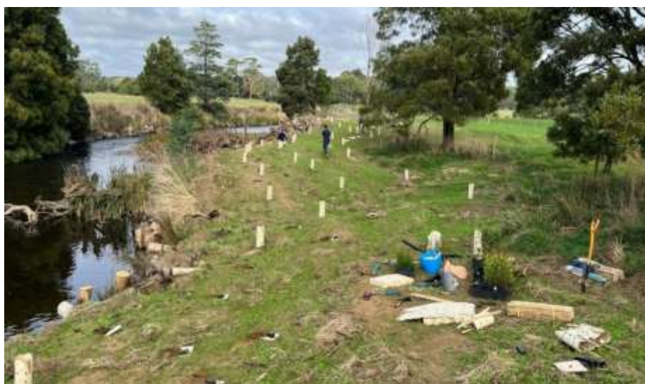
Figure 6 Inglis River capturing revegetation and timber revetment works at site 2
