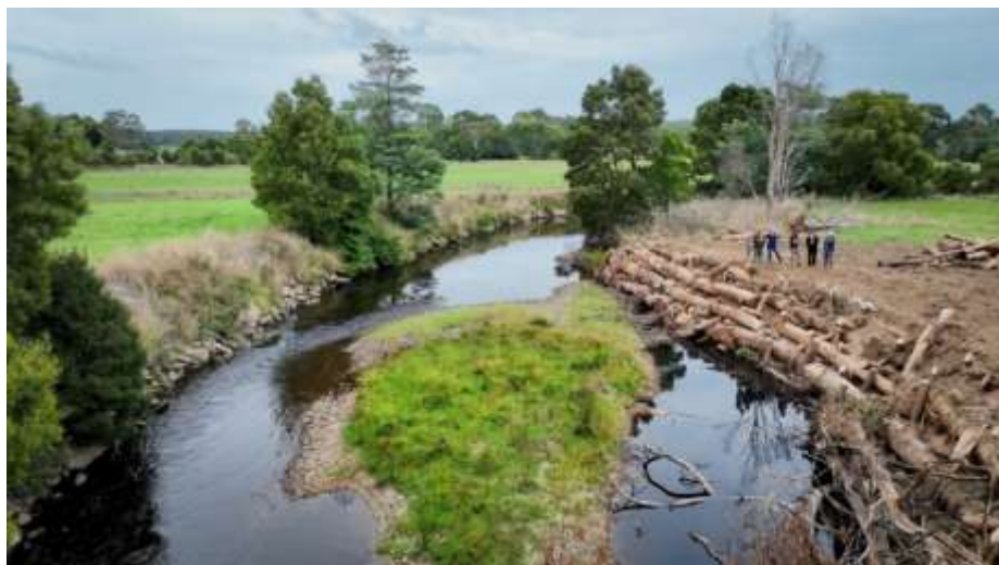
Figure 7 Inglis River capturing timber revetment works at site 2 (pre revegetation works)
