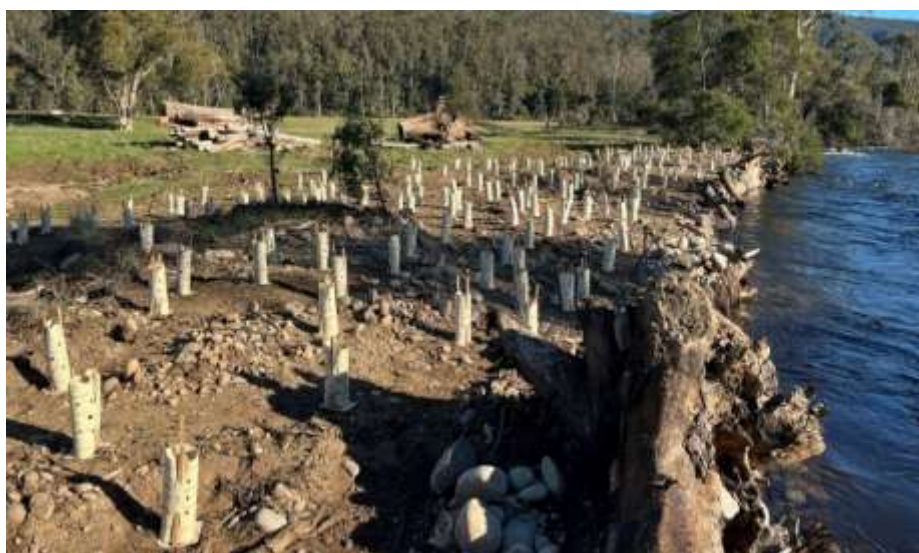
Figure 8 The Mersey River capturing timber revetment works, revegetation (fencing yet to be completed)
