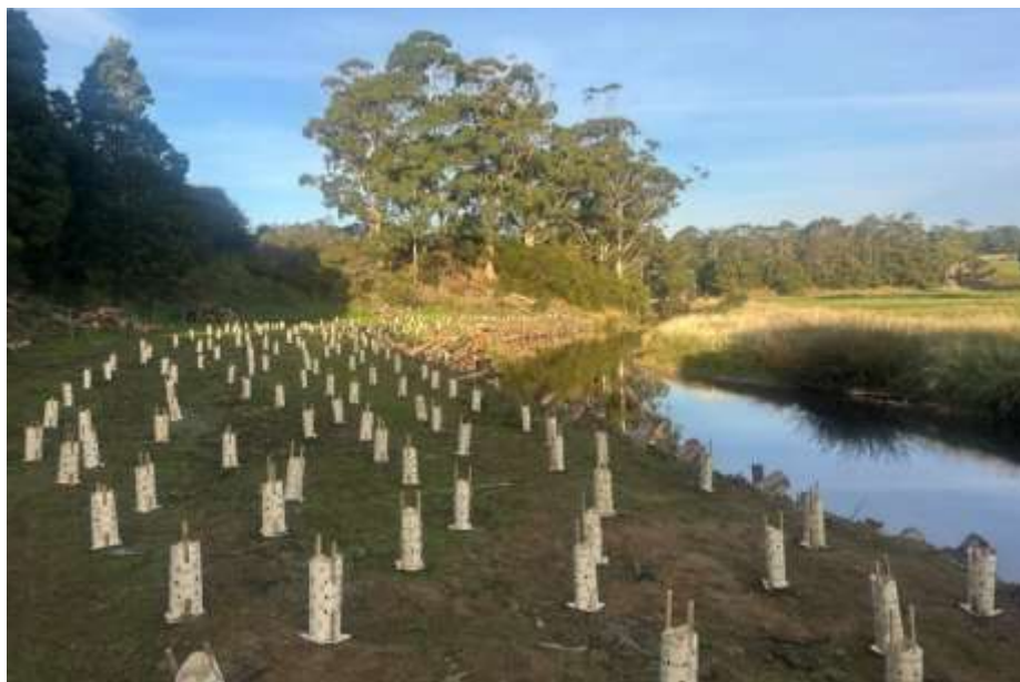
Figure 4 Inglis River capturing revegetation and timber revetment works at Site 1
