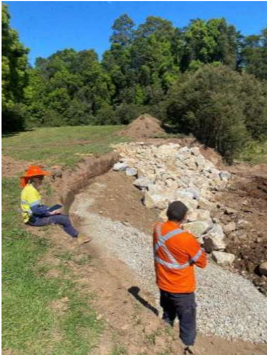
Figure 3 Granular filter with armour rock overlay, granular filter at Kennaicle Creek, Missabotti, September 2024
