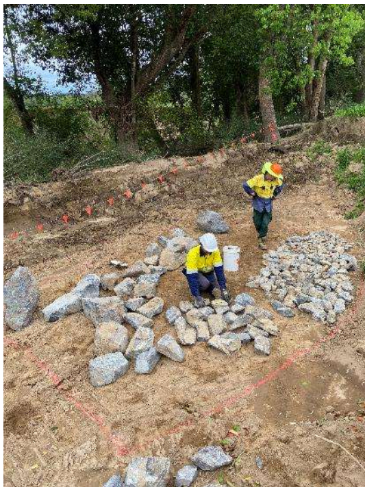
Figure 1 Sorting shot rock to test d50, Nambucca River, Bowraville September 2025
