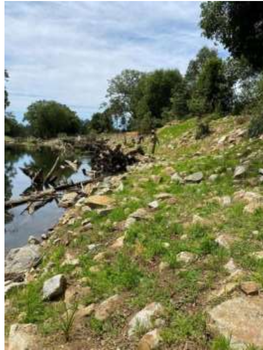
Figure 4 Soil filled revetment being planted on the Nambucca River, Bowraville November 2025
