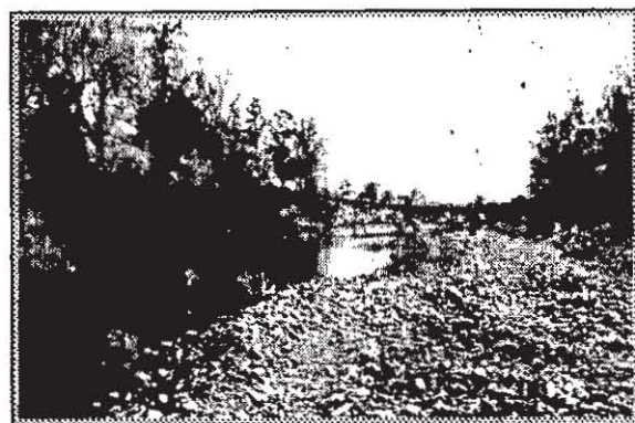
Photograph 1. BARRINGTON RIVER, GLOUCESTER, NSW, showing a section of River looking d/s from a point-bar cleared, of brush and oak to relieve flow concentration on a downstream eroding bank. This is part of the Barrington RIVERCARE plan.
