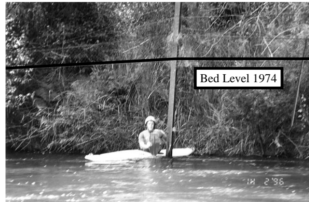
Figure 2: Hanging bottom cable of old mesh erosion control works indicating the amount of bed degradation since 1974.
