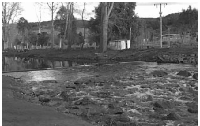
Figure 2: Rock fishway at Cowwarr knife-edge weir on the Thomson River (photo: S.Heron)
