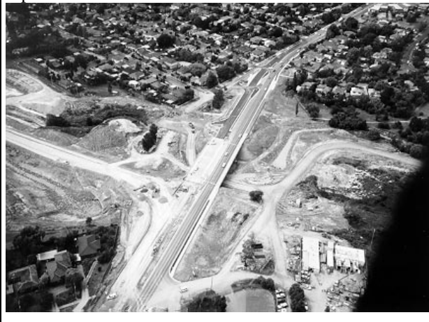
Initial stages of freeway construction - Tram Rd grade separation
