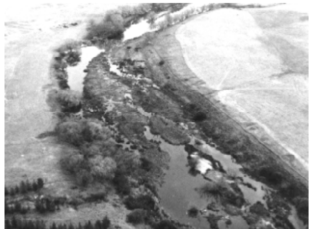
Figure 6. Aerial view of Snowy River near Dalgety 1998 showing channel contraction by formation and vegetative colonisation of in-channel bars
