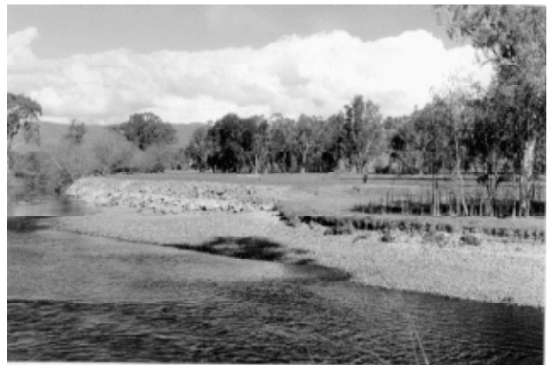
Figure 3. Tumut River at Tumut looking downstream showing rock work on bank to control channel enlargement with active bank retreat even on the inside of a bend
