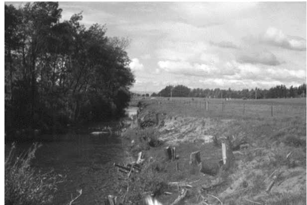
Figure 3: An example of a recommended method for removal of willows from river banks - the 'cut stump method'.
