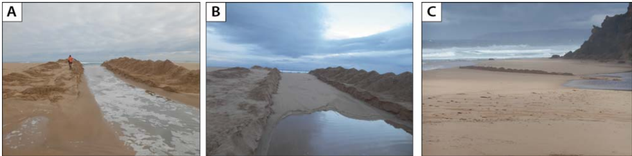
Figure 4. Second artificial opening at Aire River. (A) Day of opening. (B) Day 2: closed. (C) Day 3: full infill.
