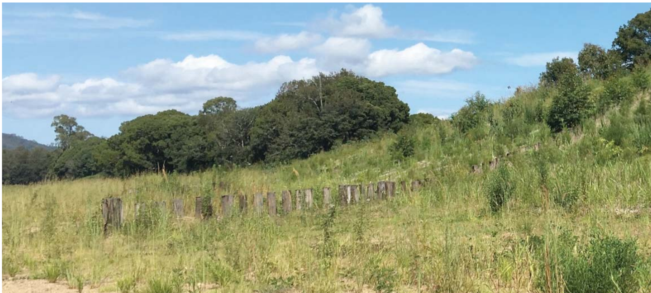
Figure 5. Post works - Mary River, Kenilworth (view looking upstream 26/03/2016)
