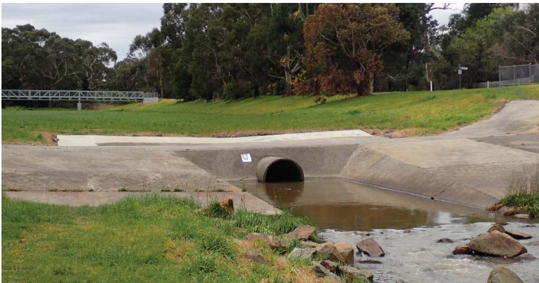
Figure 3. Dandenong Creek showing the existing low-flow pipe outlet and grassed high-flow channel
