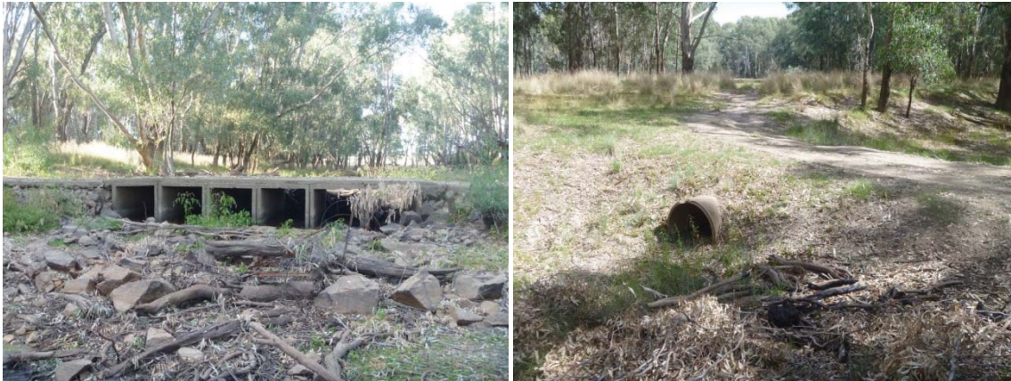
Figure 1. Raised track crossings with box culverts (left) and pipe culvert (right)
