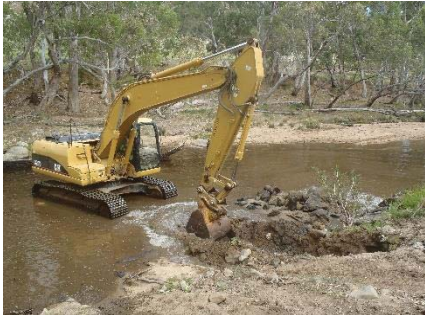
Figure 12a. Trench dug into bank for desired alignment.
