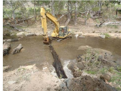
Figure 12b. Length/s of wood placed in trench at desired angle.
