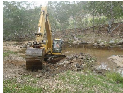
Figure 12d. Trench filled in with soil and compacted.
