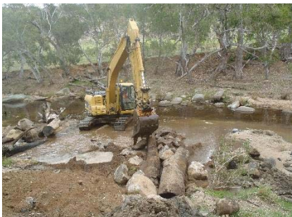
Figure 12c. Anchoring rock placed on and around wood.
