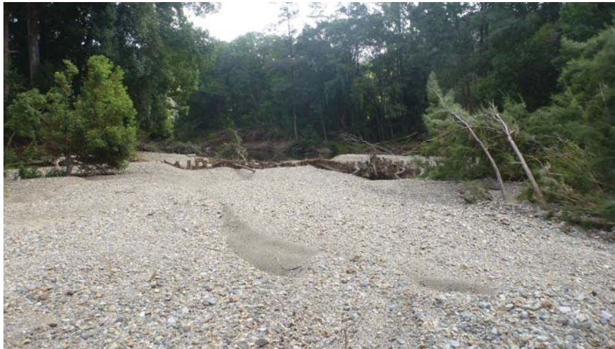
Figure 11: View upstream through the river left flood chute of the lower cutoff channel (3 February 2012). The photo shows gravel aggradation upstream of a series of timber pin rows constructed at 0.9m above natural surface. The timber pins in the foreground were subsequently buried during a flood event one week later and an additional pin row was installed in late 2012 between these two rows, resulting in further aggradation and elevation of the incised flood chute following 2013 floods.
