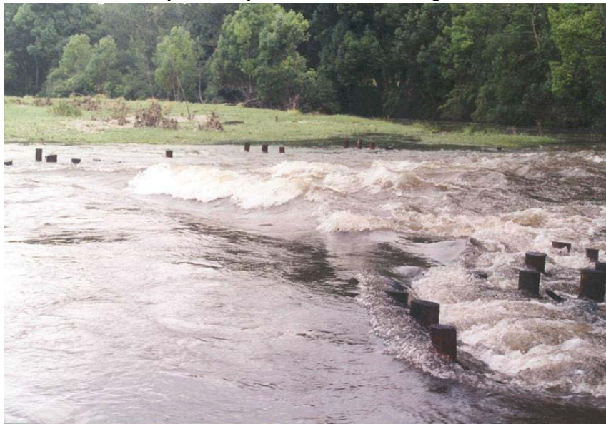
Figure 2: Elevated Log sill (ELS1) with timber pin radials, Orara river with approx 0.6m flow depth above the ELS. Note the influence of timber pins on upstream backwatering and wave formation downstream.
