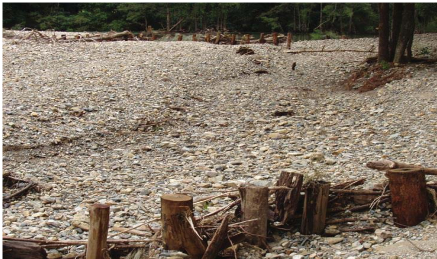
Figure 11: View upstream through the river left flood chute of the lower cutoff channel (3 February 2012). The photo shows gravel aggradation upstream of a series of timber pin rows constructed at 0.9m above natural surface. The timber pins in the foreground were subsequently buried during a flood event one week later and an additional pin row was installed in late 2012 between these two rows, resulting in further aggradation and elevation of the incised flood chute following 2013 floods.
